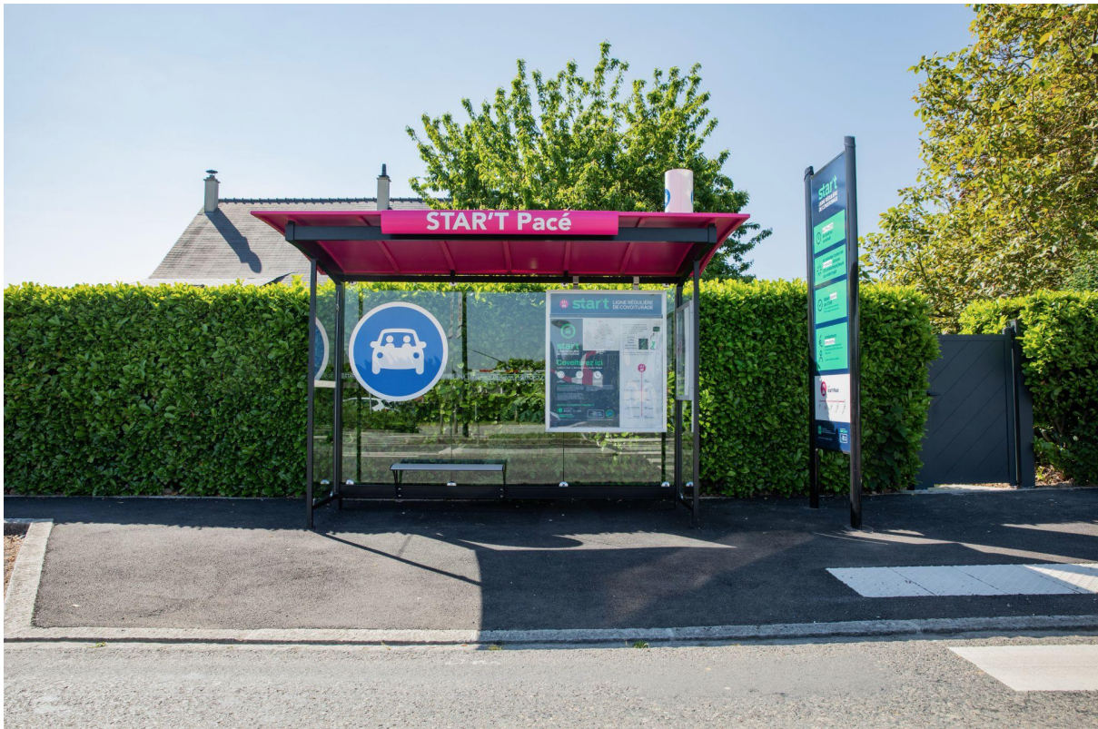
Carpooling stop on a line located in the suburbs of Rennes, France.
